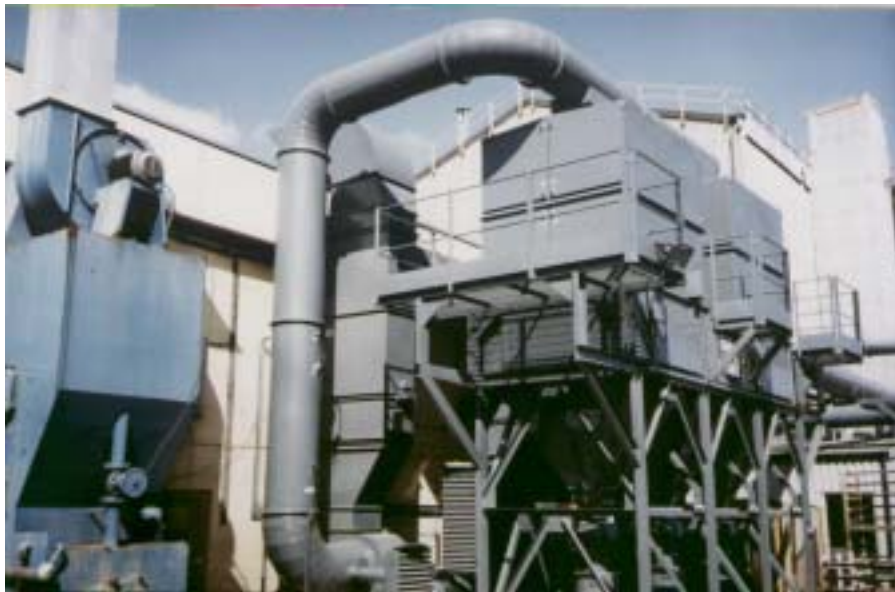
The emission monitoring system installed to monitor bagfilters at an iron foundry
